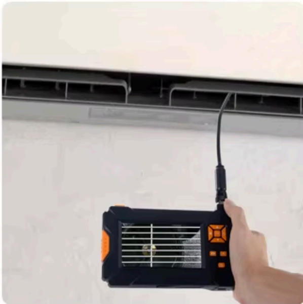
Air condition inspection
